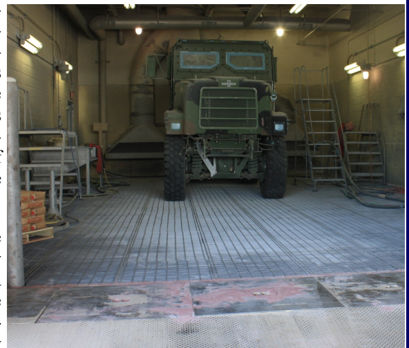
Figure 1. Photo of the interior of the blast booth at Camp Lejeune, NC with a vehicle ready to be abrasive blasted.
